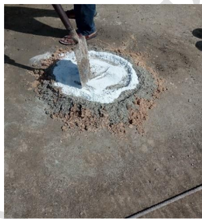
(b) Cement and recycled glass powder added to fine aggregates
