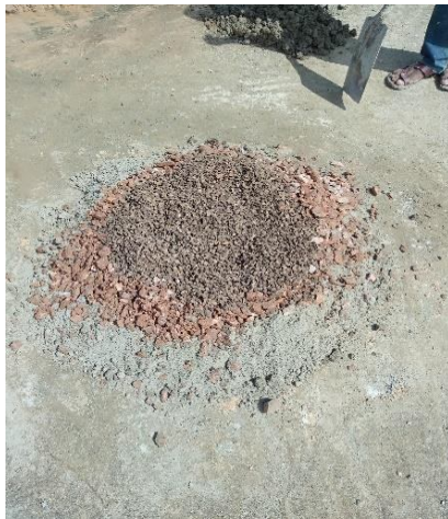
255 (d) Coarse aggregate and Palm 256 kernel shells added to the mixture 257 of cement, recycled glass palm 258 powder and fine aggregate
