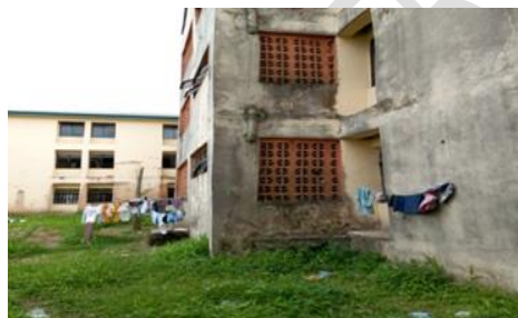
Plate 2: Showing condition of building in Crutech
