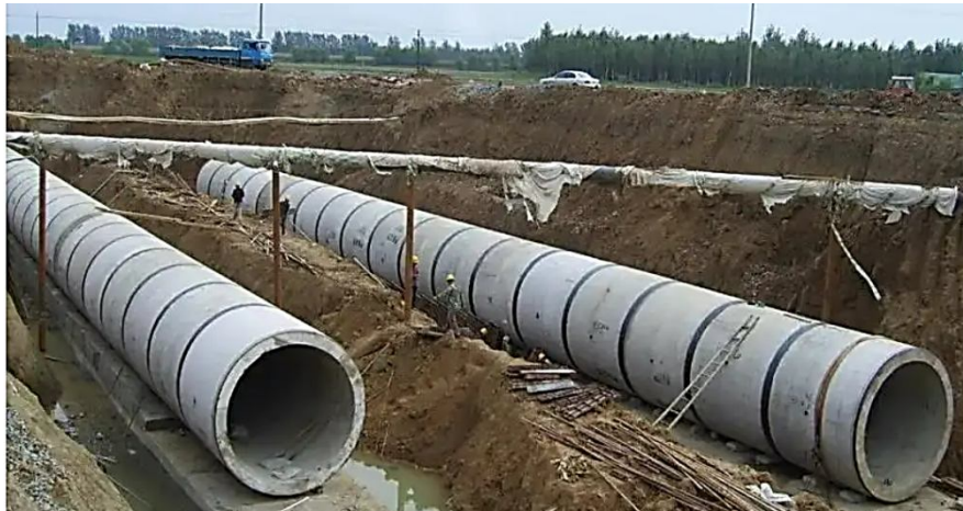
Fig.1. Hydroelectric power station pressure piping
