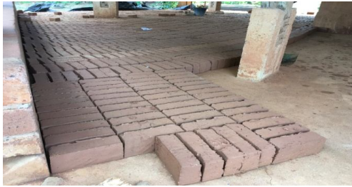
Fig. 6. Natural drying of bricks
