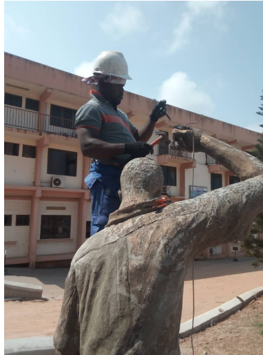
Fig. 4. Passing of electric wire and fixing of the bulb
