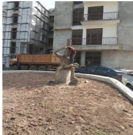
Fig. 2. Finishing with cement mixture and clearing of surroundings
