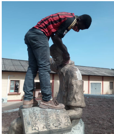
Fig. 1. Surface preparation of the outdoor concrete statue
