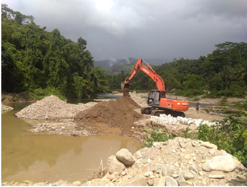
Fig 4: The bulldozer collecting sand from the middle of the river.
