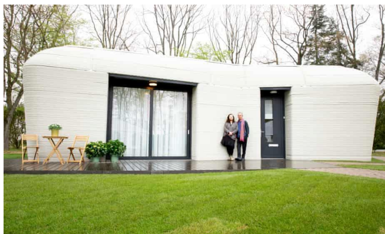
Figure 3. 3D-printed house in Eindhoven, Netherlands [9].
