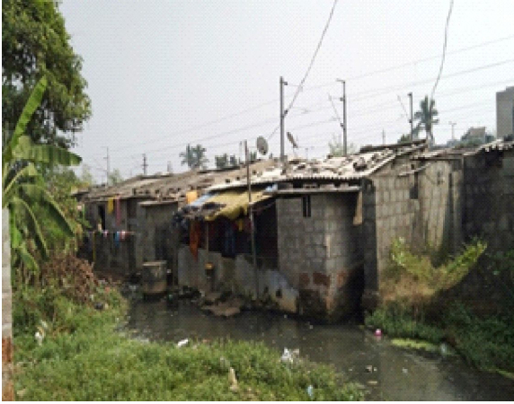
Fig 2(a): No proper drainage facilities
