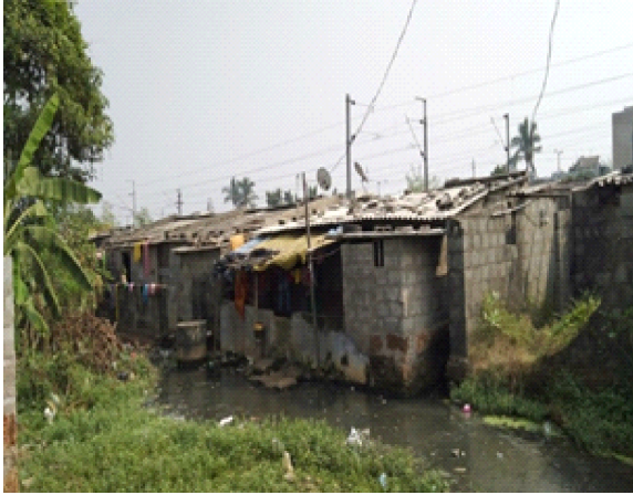
Fig 2(a): No proper drainage facilities
